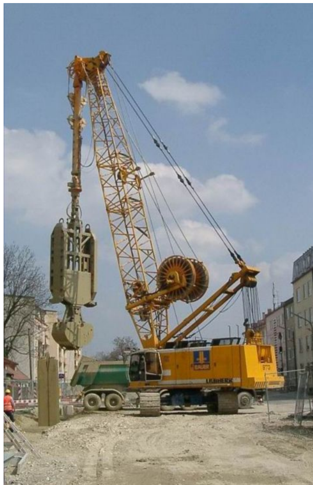
Fig. 16 Diaphragm wall preparation during the construction of the Munich subway
